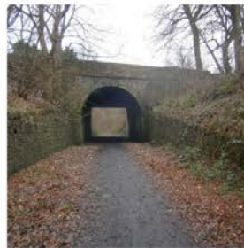
4 Underbridge at A80
