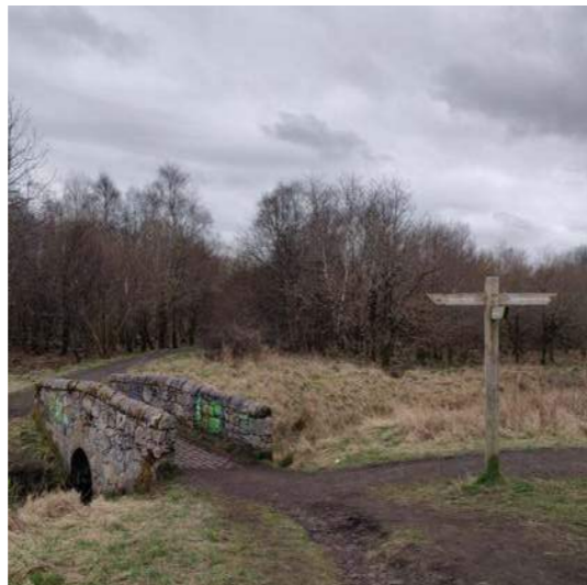
12 Footbridge to Core Path 83, and East towards Core Path 84
