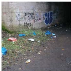
5 Littering along the underbridge
